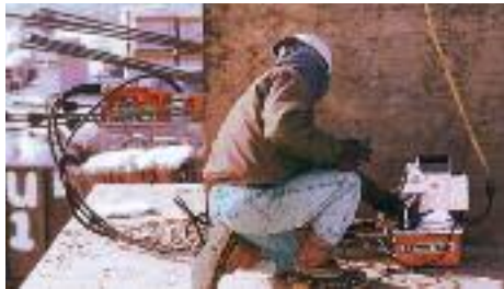
The PE60 used for pre-stressing.
